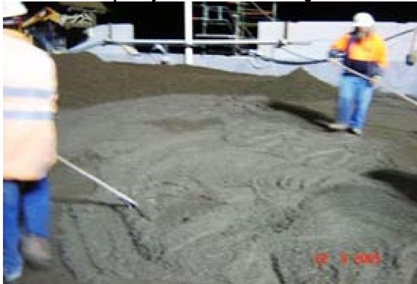
PICTURE 3. Damaged surface is blown and Completely covered with bedding mix
